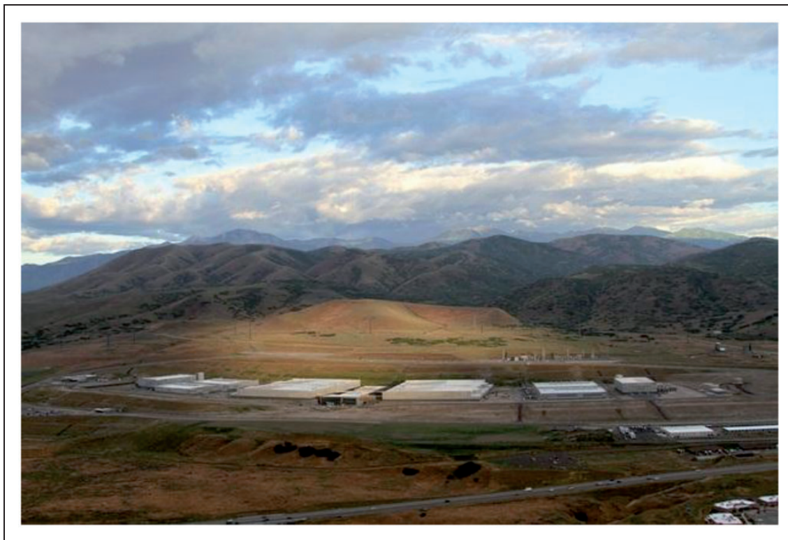
Figure 1. EFF public domain image of NSA Utah Data Center 2013 (Higgins, 2014).
